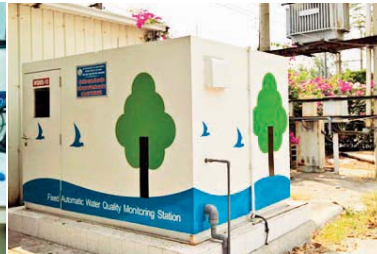
Automatic monitoring system that measuring after-treated water quality
