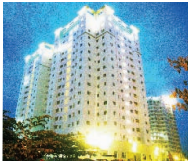
Nhat Lan 3 Apartment Building
